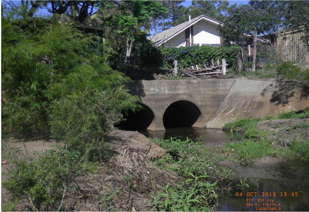
Graduate Street culvert looking upstream
