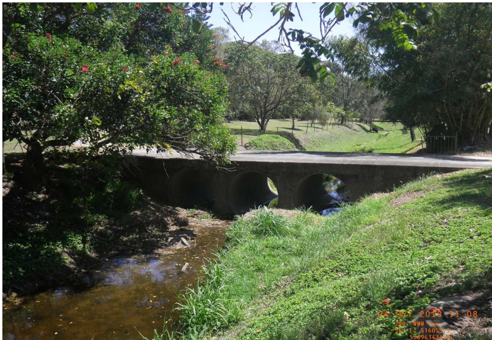
Haig Street private property culvert looking downstream
