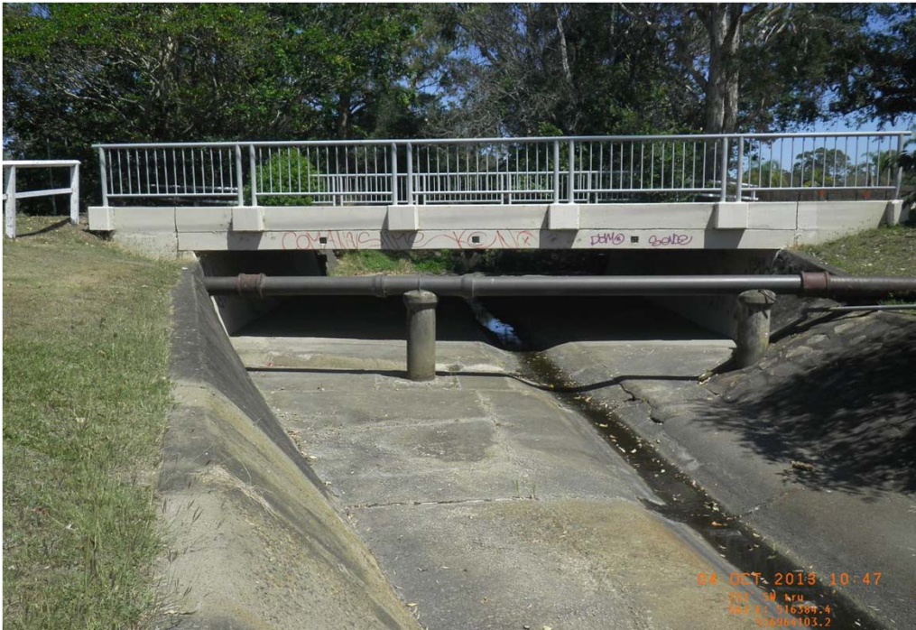
Stradbroke Avenue looking upstream
