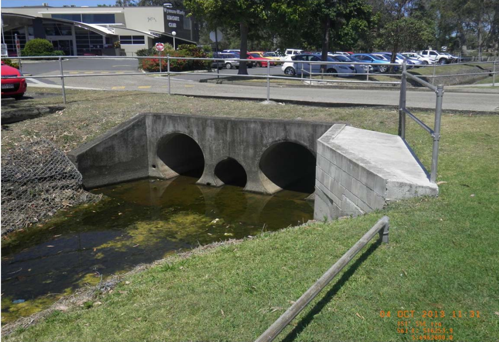
Wynnum Mainly League Club Access Road Looking Upstream
