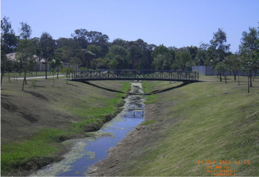
Robtrish Road footbridge looking downstream
