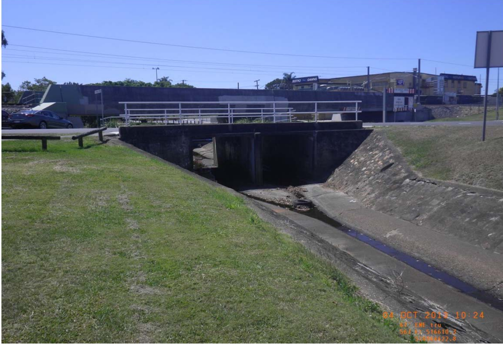
Daisy Street culvert looking downstream
