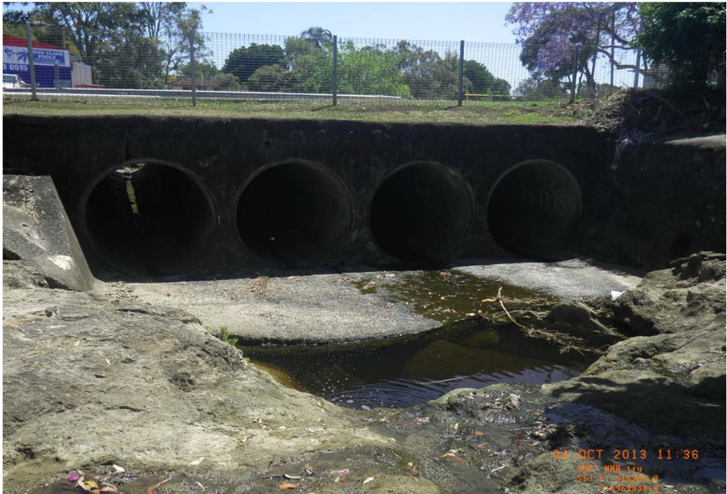
Wondall Road culvert looking downstream
