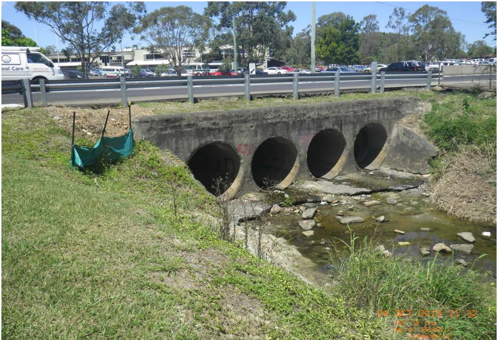
Wondall Road culvert looking upstream
