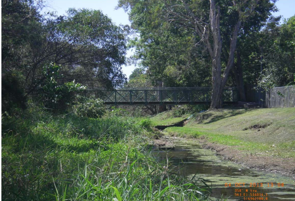
Barbara Street footbridge looking downstream
