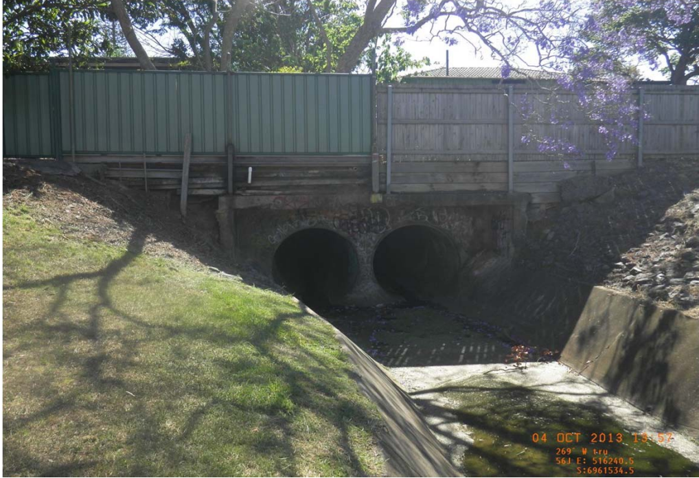
Graduate Street culvert looking downstream
