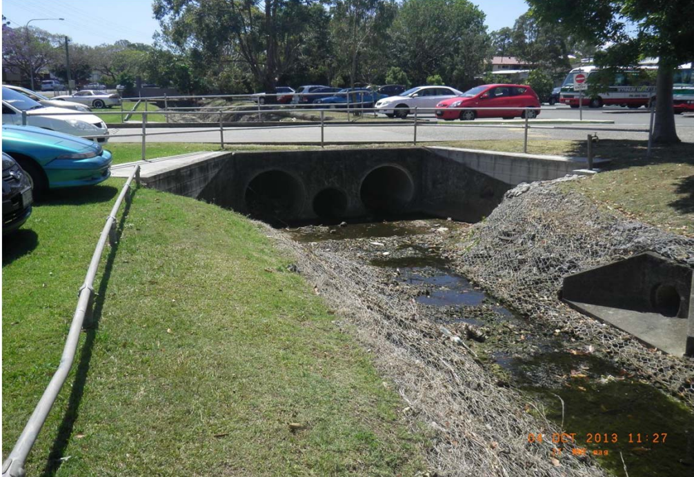
Wynnum Mainly League Club Access Road Looking Downstream
