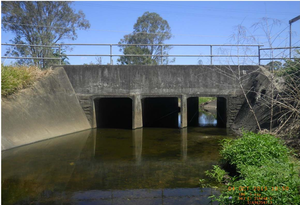
Stannard Road culvert looking upstream
