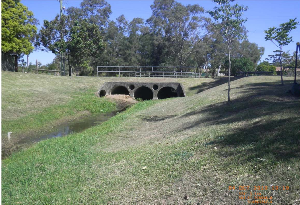
Radford Road culver looking upstream
