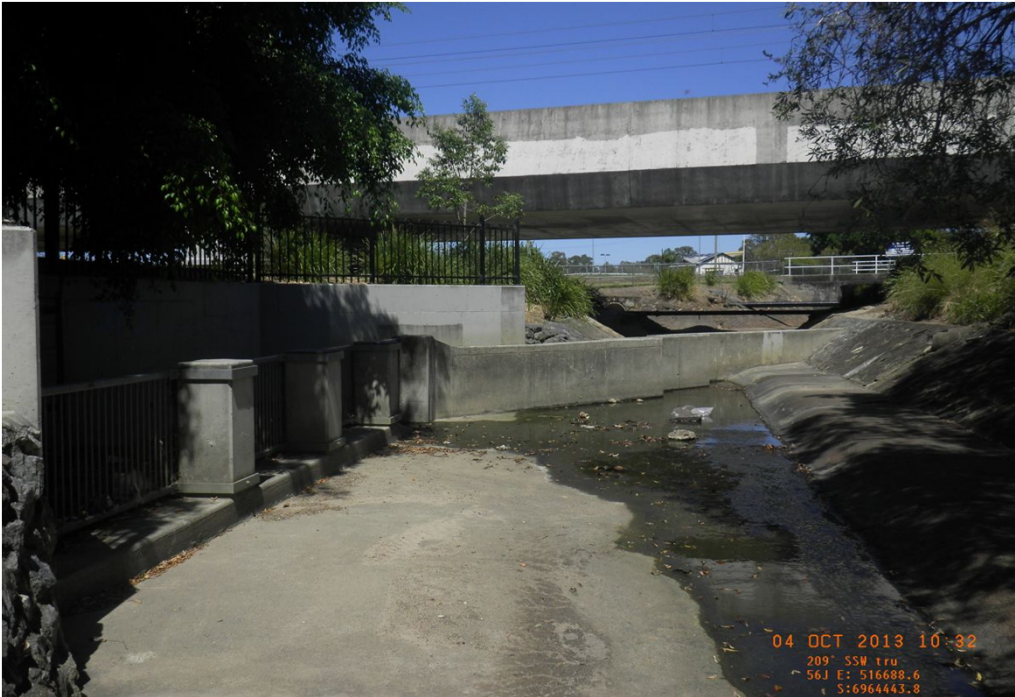
Queensland Rail bridge looking upstream
