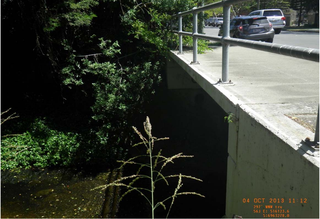
Preston Road bridge looking downstream
