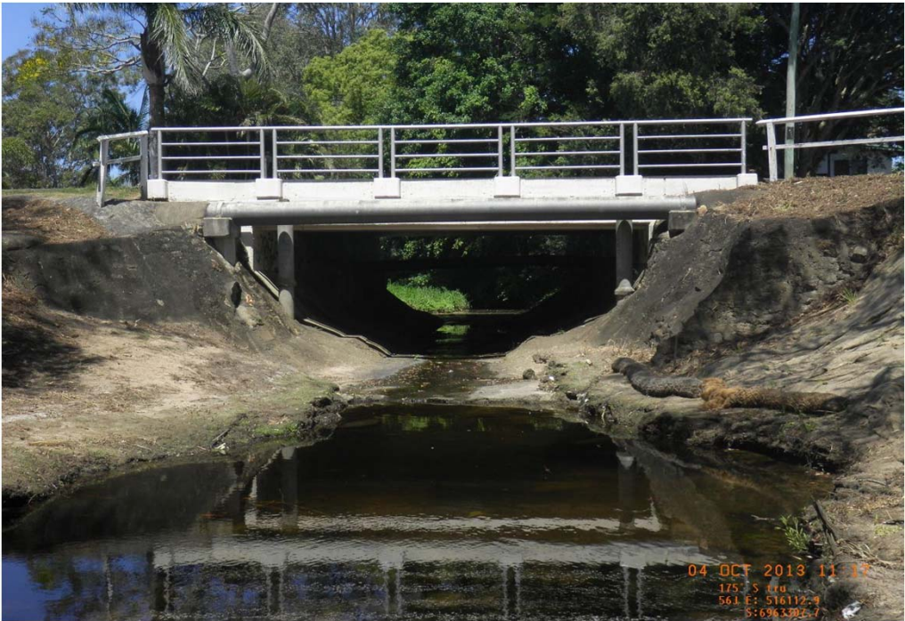
Preston Road bridge looking upstream
