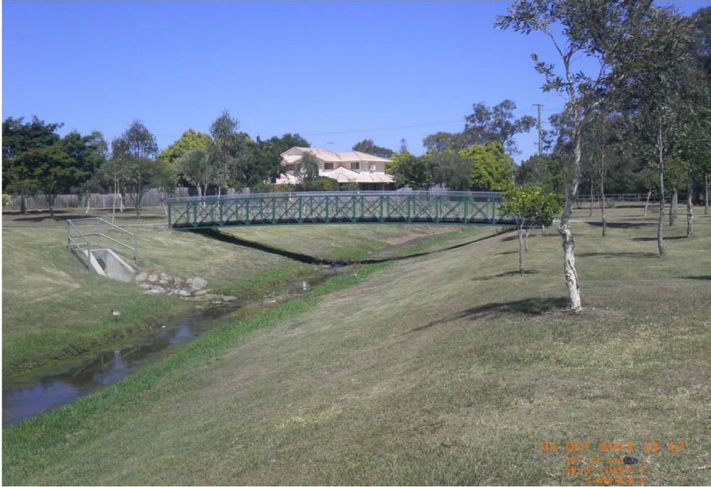
Robtrish Road footbridge looking upstream
