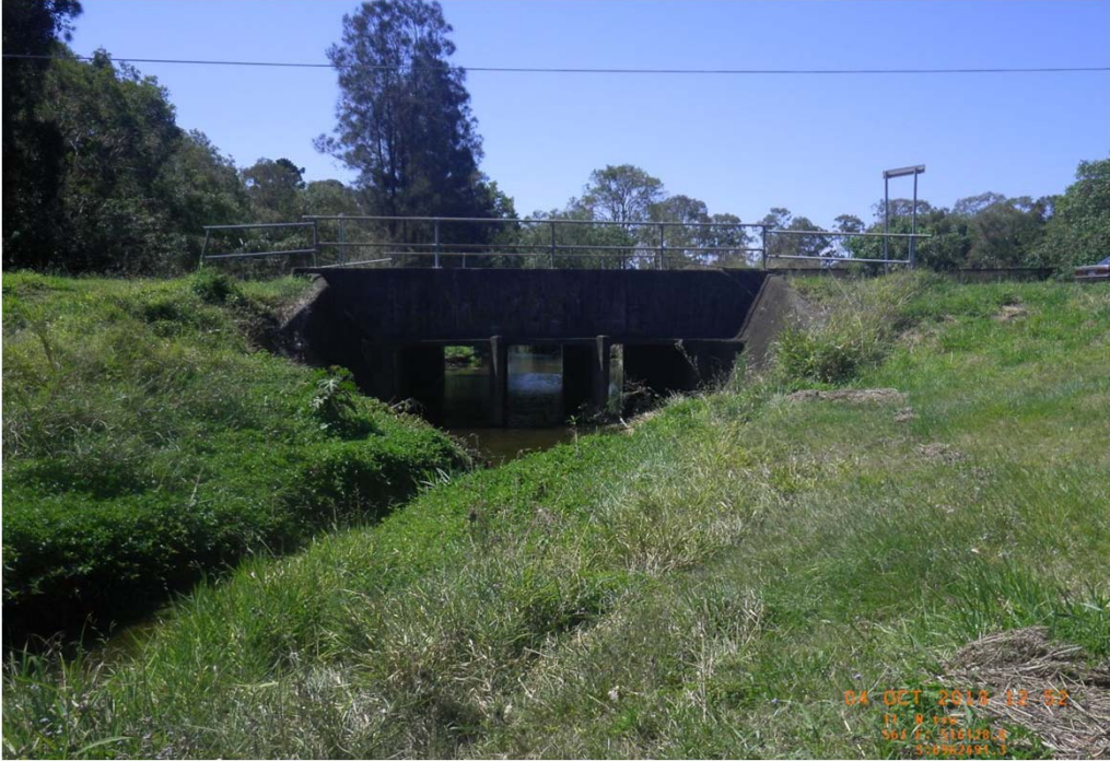
Stannard Road culvert looking downstream
