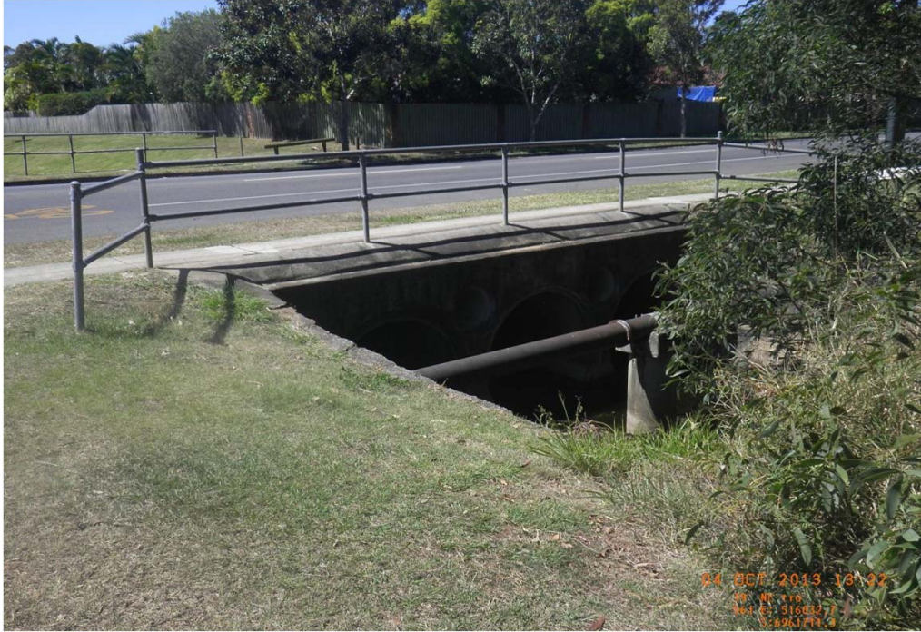
Radford Road culvert looking downstream
