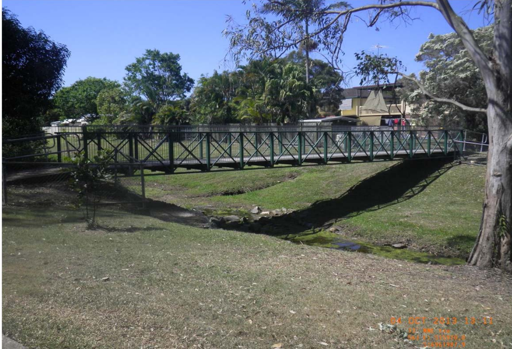
Talwong Street footbridge looking downstream
