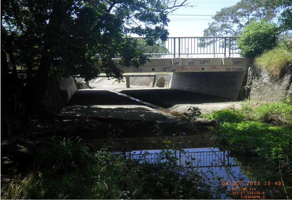
Stradbroke Avenue looking downstream
