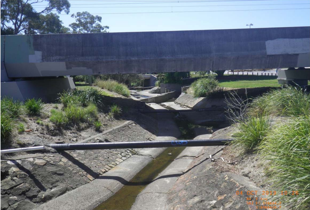
Queensland rail bridge looking downstream
