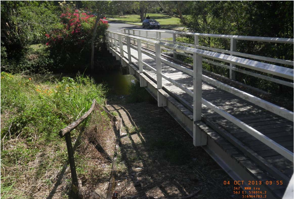
Coreen Street footbridge looking from right hand bank from upstream side
