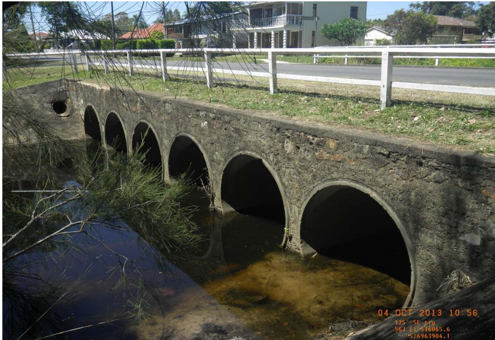
Chandos Street culvert looking upstream
