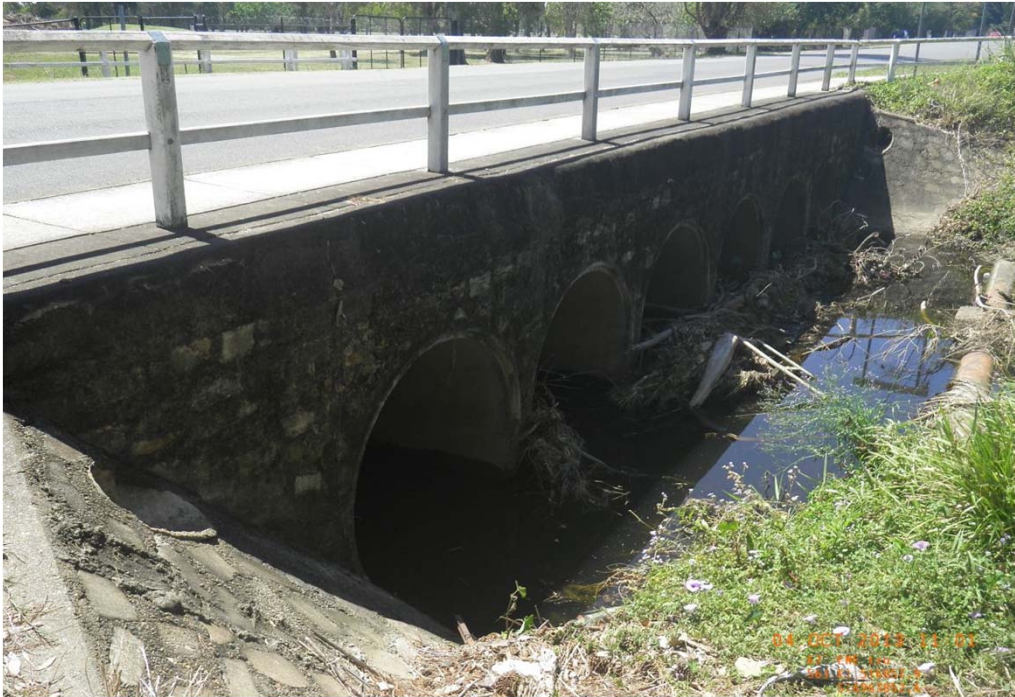
Chandos Street culvert looking downstream
