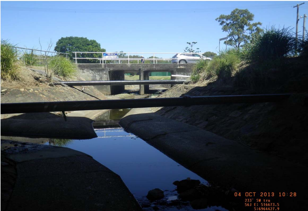
Daisy Street culvert looking upstream
