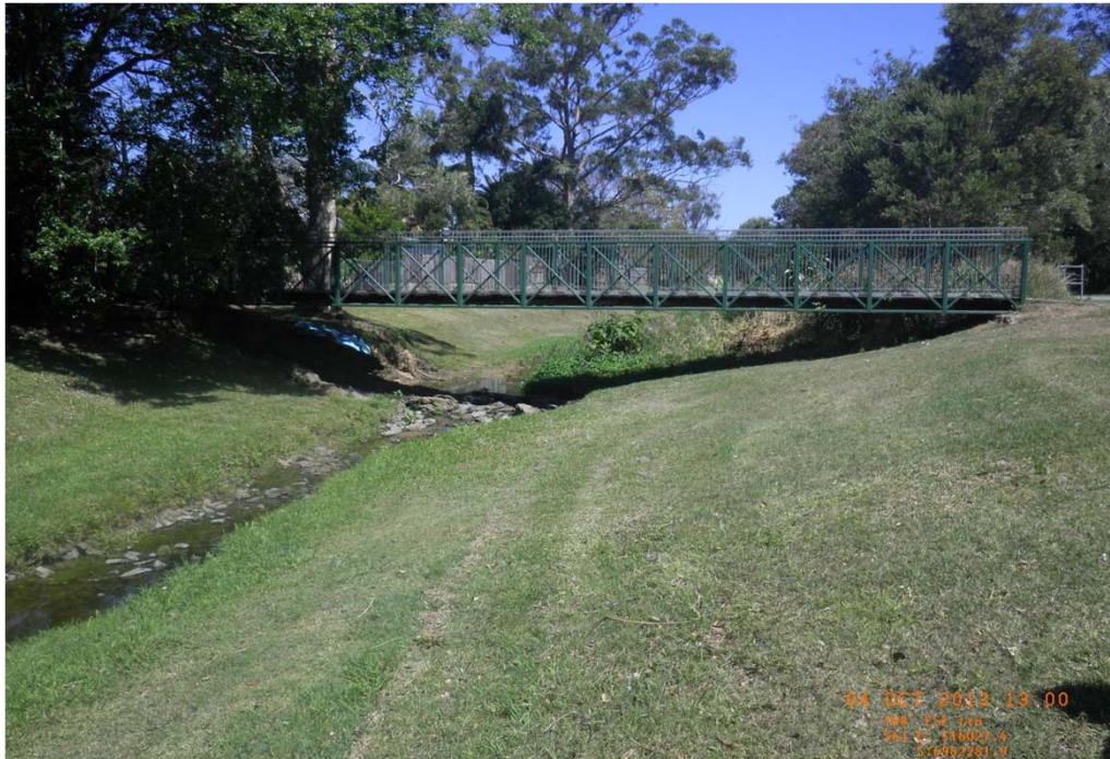
Barbara Street footbridge looking upstream
